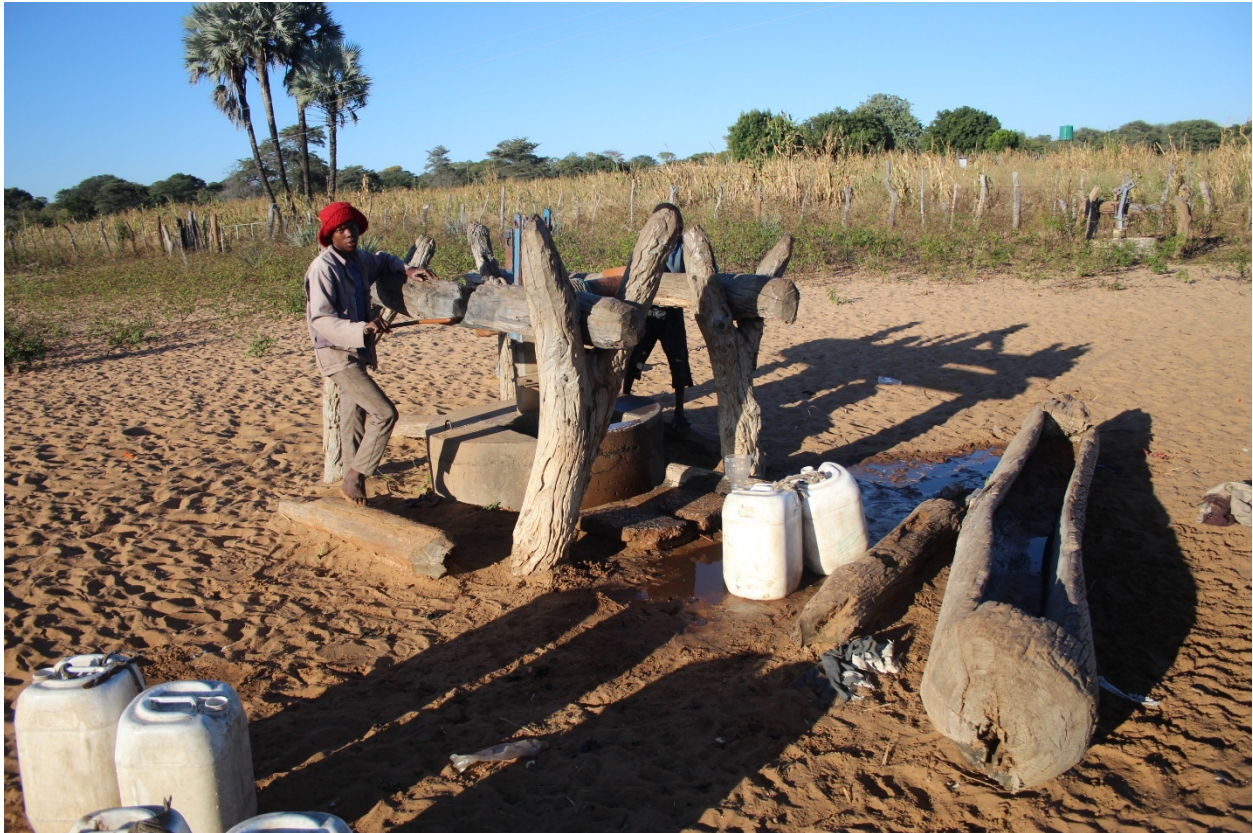
Figure 5: The existing traditional well in Oluwaya that will be upgraded to a modern well (Authors 2025).
