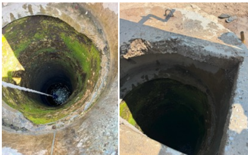
Figure 5-4: Safety risk – uncovered community well
