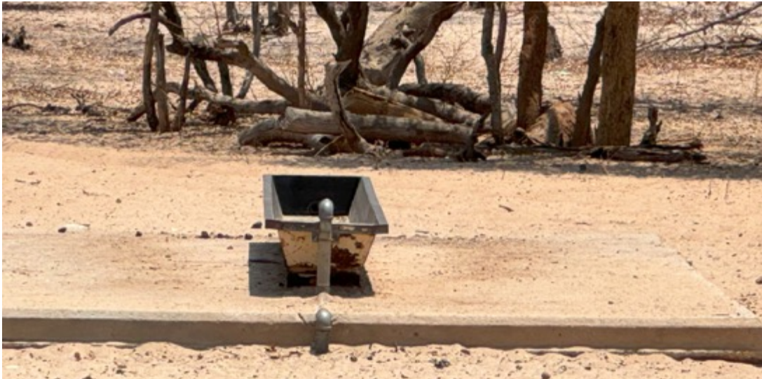
Figure 5-9: Properly constructed Livestock trough with a concrete platform – Oluwaya water point
