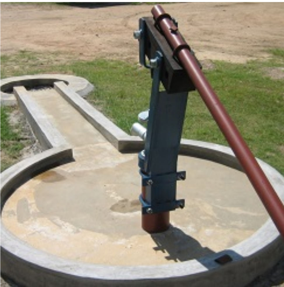
Typical sanitary seal
