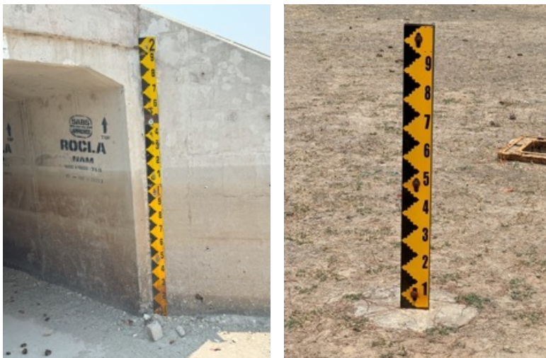
Figure 5-21: Water Level Measuring Scale at A Road Culvert in Oshanalumono (TEC, 2024)
