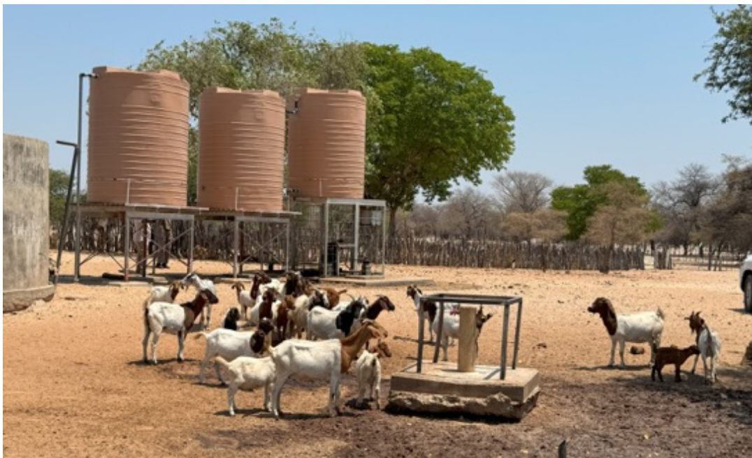
Figure 5-8: Oluwaya water point has good infrastructure, however – the borehole has saline water and it is not fit for human consumption – basic water purification is required)
