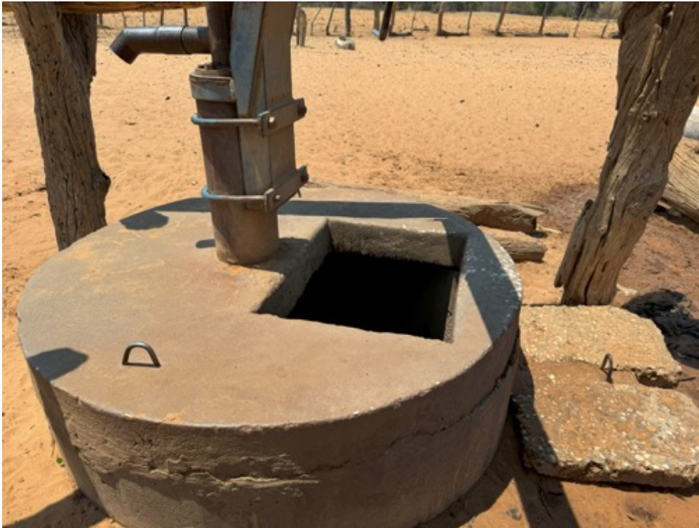
Figure 5-10: Detailed Well infrastructure- Oluwaya village
